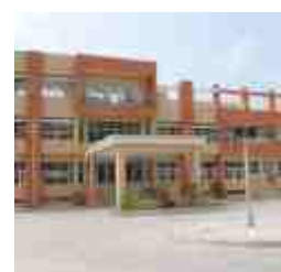
Water Supply and Sanitation Department Patilala
