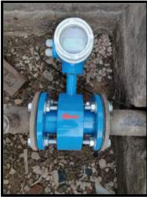
Photographs of Electromagnetic flow meter provided at water supply line and STP outlet
