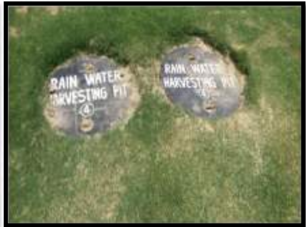
Rain Water Recharging pits provided within the project premises
