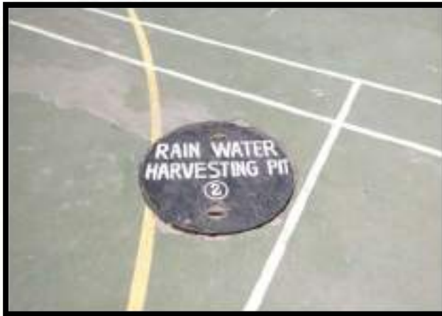
Rain Water Recharging pits provided within the project premises
