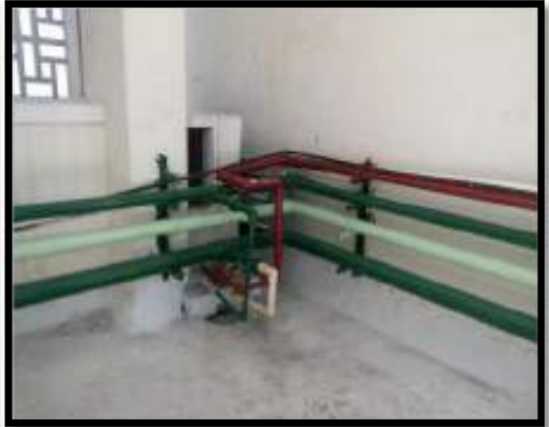
Photographs showing STP & Colour Coding of the pipelines
