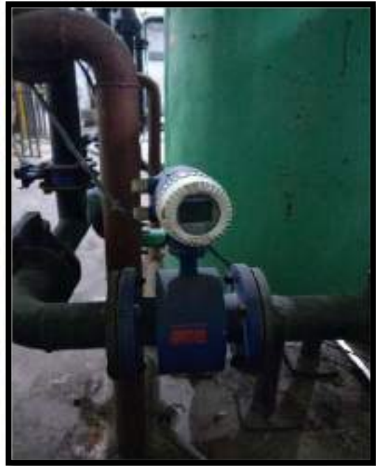
Photographs of Electromagnetic flow meter provided at water supply line and STP outlet
